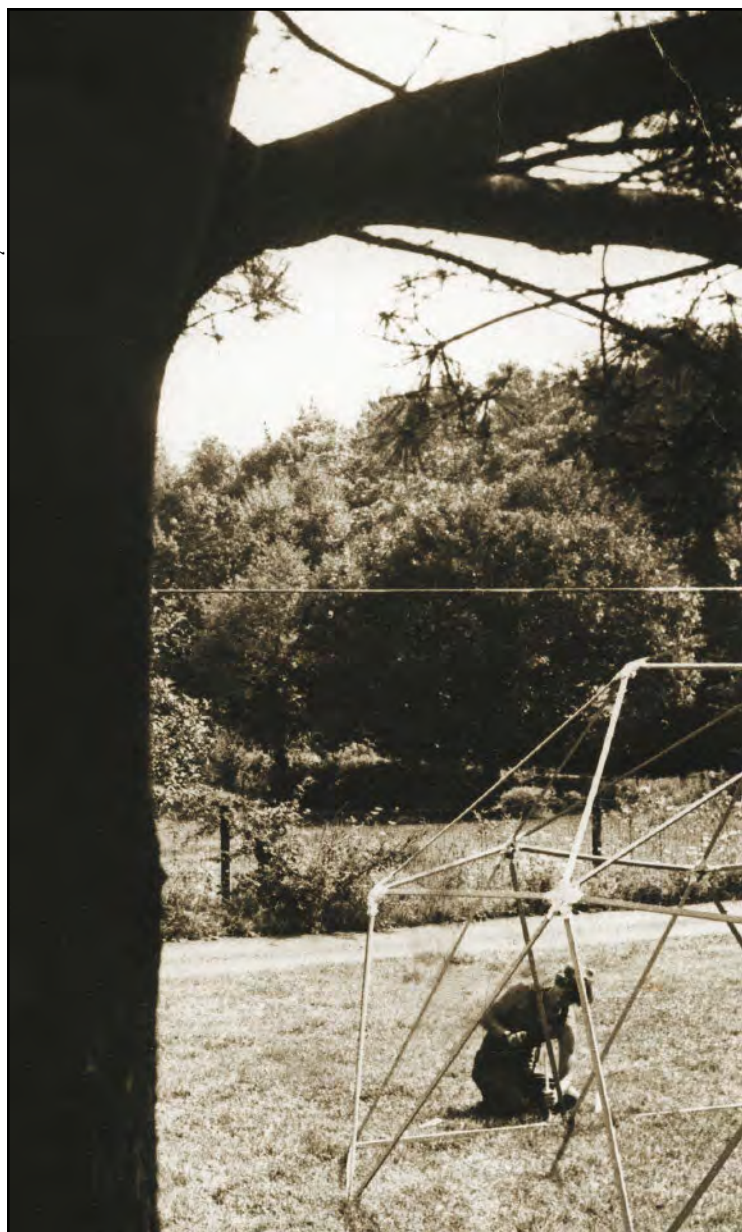
25' test for Kirkridge Dome with metal strapping hinges.
